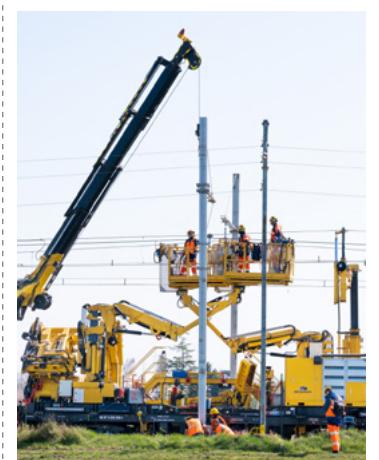
TSO train renewing overhead lines in the 1,500 volt network
