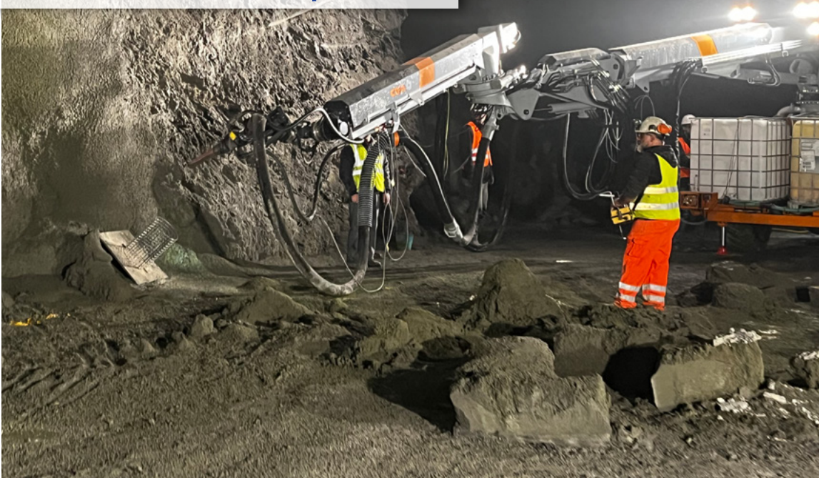
Mamba shotcrete pump in use in a tunnel
