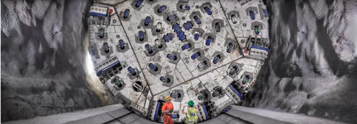
Start of tunnelling at the Brenner Base Tunnel
