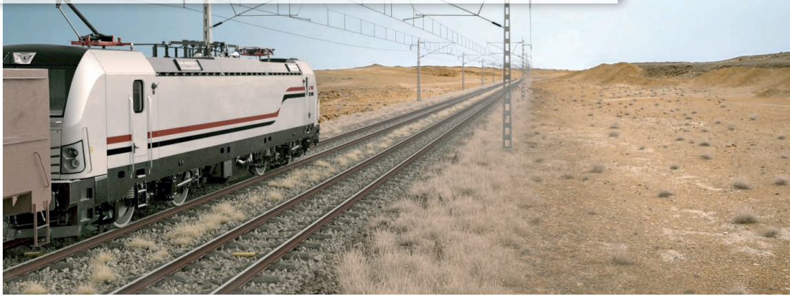
The first 660 of a total of 1,800 kilometres of track have now been contracted.
